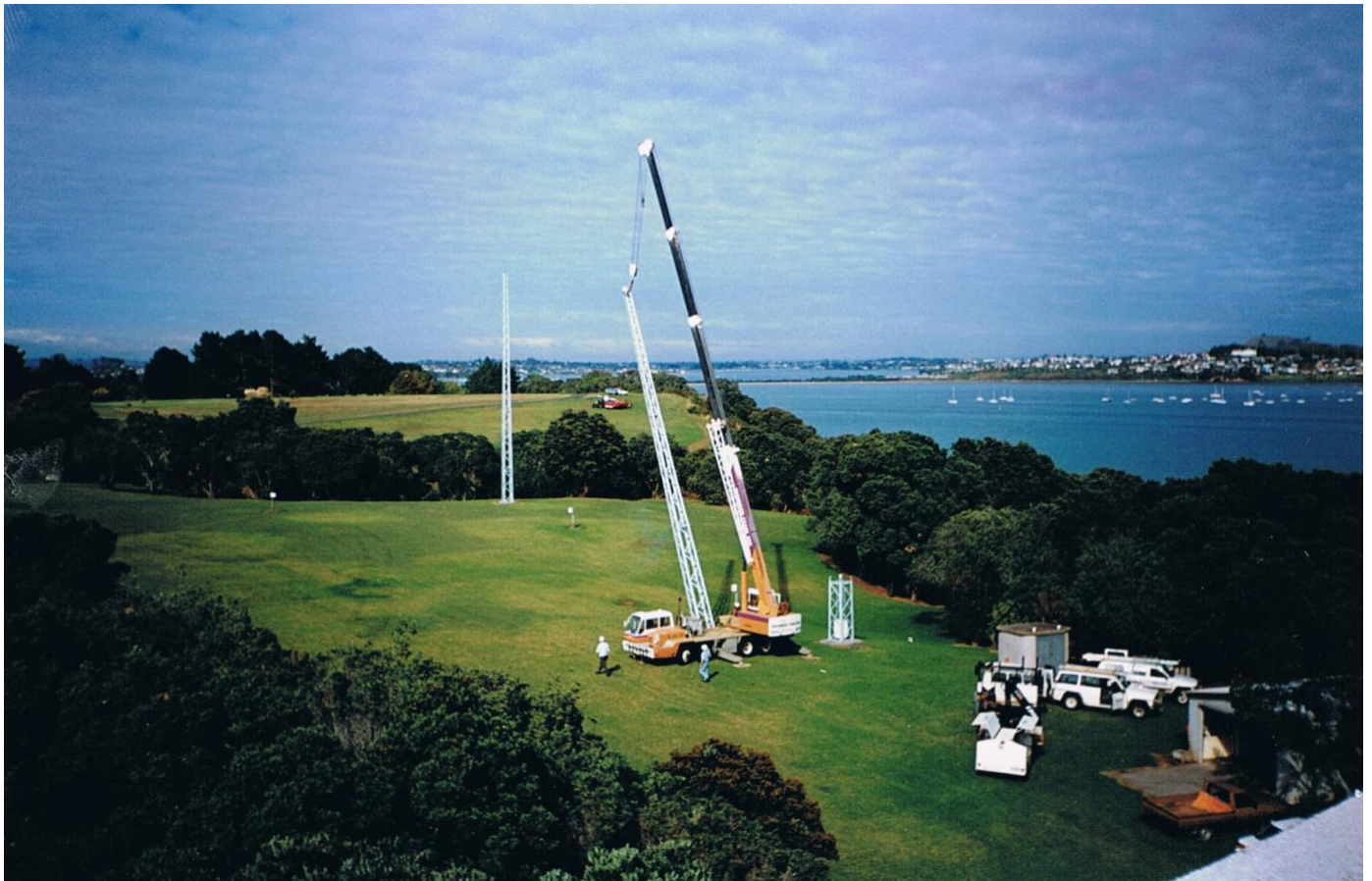
Lowering the towers at ZLD, 1993. The end of an era.
